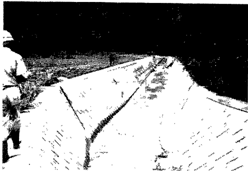
Photo. 6. Slightly damaged revetment in the Aokawa River.
