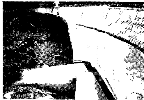
Photo. 6. Slightly damaged revetment in the Aokawa River.
