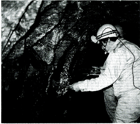
Photo. 1. Headrace tunnel without concrete lining. (Shimo-Nishitani run of the river hydropower station, Chugoku Electric Co. Ltd.)
