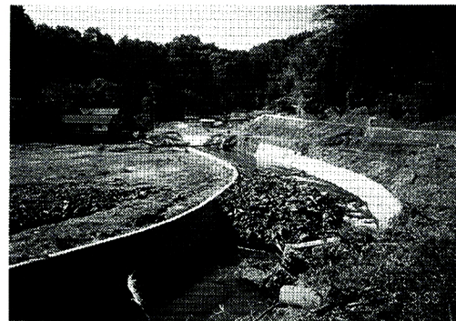
Photo. 4. Sedimentation in a curved channel of the Takimizu River.
