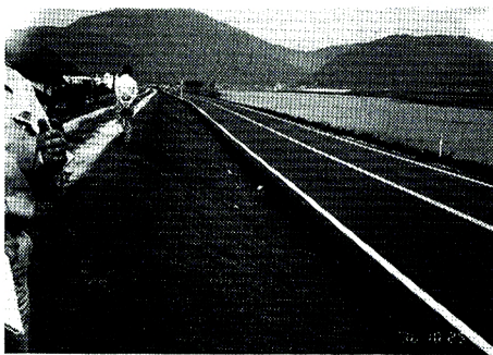
Photo. 4. Temporary levees in the downstream reach, about 10 km from the river mouth, of the Maruyama river. (Notice white garbages on the bank slope indicating the highest flood level mark)
