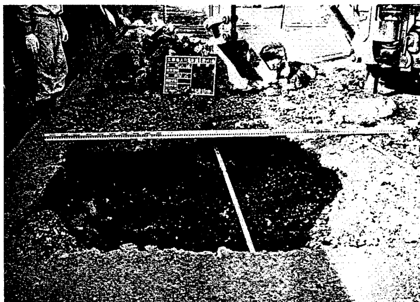
Photo. 1 Cavitation under the pavement behind revetment.
