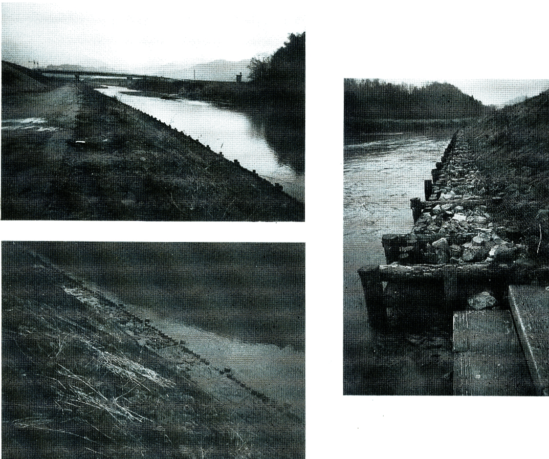
Photo. 3 Revetment as a kind of rich-in-nature river improvement works in the Izushi river, a tributary of the Maruyama river, Hyogo prefecture.
