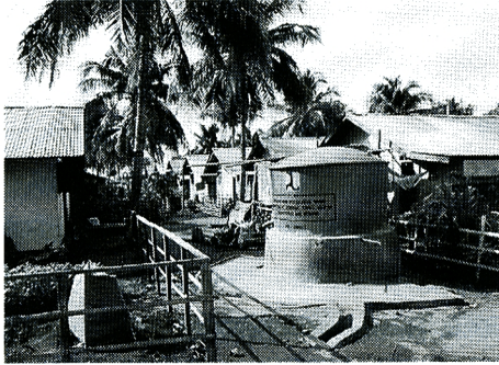
Photo 11 Water tank at Uring Baru
