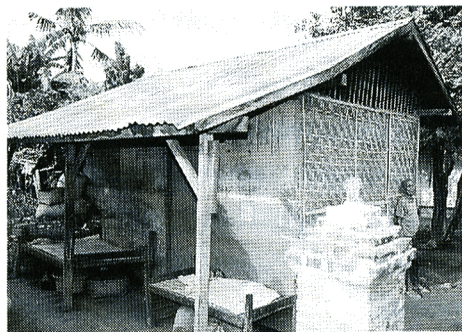
Photo 4 Restoration house at Kalianget village
