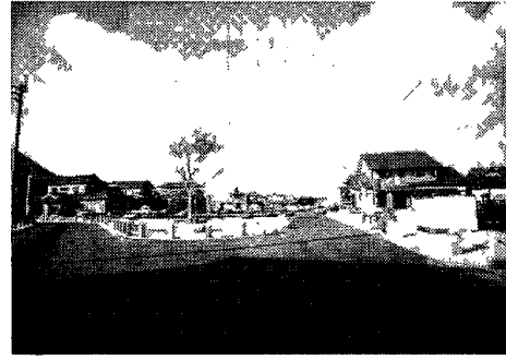
Photo 3. Rebuilt houses at a resettlement site
