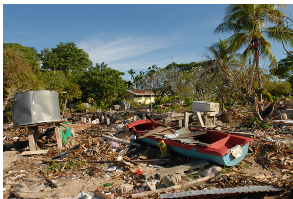
Photo 2 Damage at Marakerava Village, Gizo Island (May 27, 2007)
