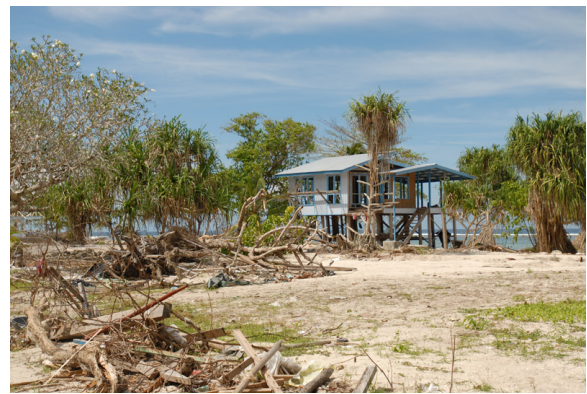
Photo 1 Damage at Titiana Village (May 27, 2007)
