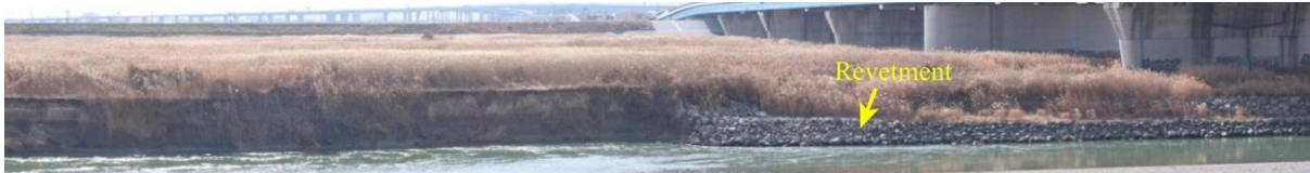
(A) A section of natural bank that extends upstream of the section protected with revetment
