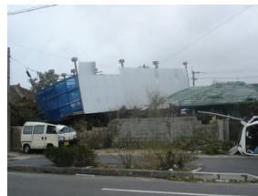
Photo 15 Lightweight steel storehouse got upon the neighbouring house
