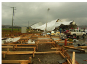
Photo 18 Remained wooden foundations of a lightweight prefabricated house
