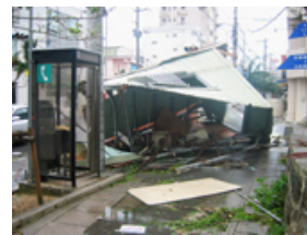
Photo 16 Lightweight prefabricated house blocked the road broke a telegraph pole
