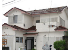
Photo 11 Openings prevented by shutter
