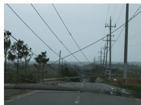
Photo 19 Telegraph poles blocked the road
