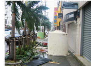
Photo 5 Fall down of water tank
