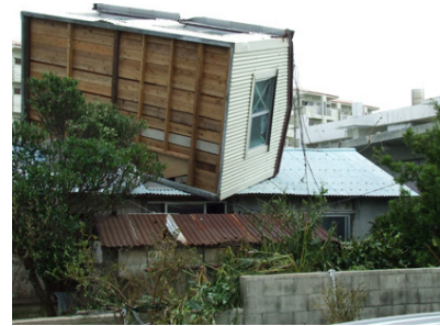
c. Lightweight prefabricated house got upon the neighbouring house.
