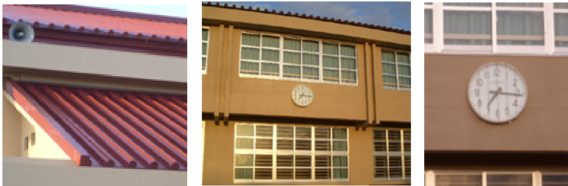
a. Well maintained roofing. b. Openings installed partitioned sash with thick glass. c. Clock protected with lattice.
