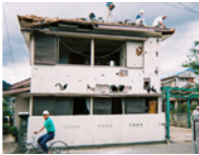
a. Broken walls and openings. b. Break on lightweight concrete wall. c. Falling down of concrete wall.
