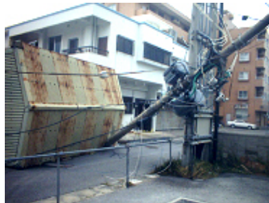
Photo 15 Lightweight prefabricated house broke a telegraph pole. (Ishigaki city office presents)
