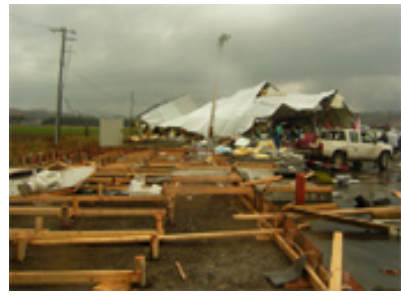
Photo 16 Remained wooden foundations of a lightweight prefabricated house. (Hokkaido kaihatu office presents)
