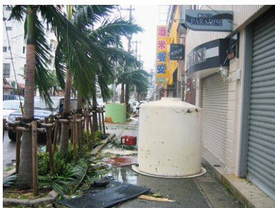
Photo 10 Water tank fell down from the roof. (Ishigaki city office presents)
