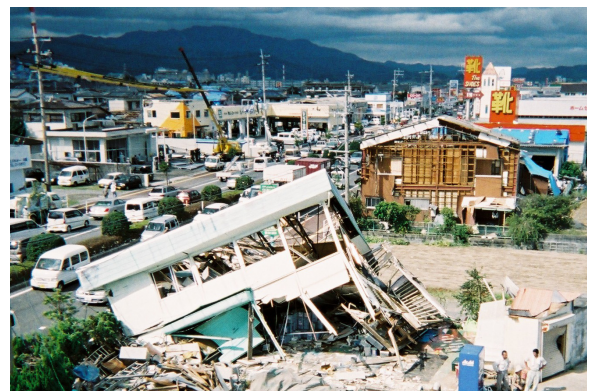
Photo 2 Collapsed houses on the track of tornado.
