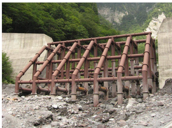
Photo 1 A grid dam constructed to prevent downstream sediment disaster of debris flow at Hirayu River, Gifu Prefecture, Japan
