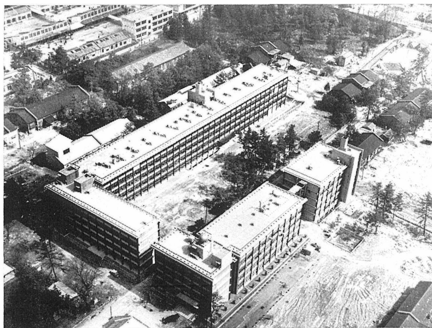
The Institute under construction in Uji
