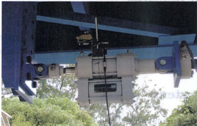
Photo 2.2: Photo of the Attached Damper Specimen
