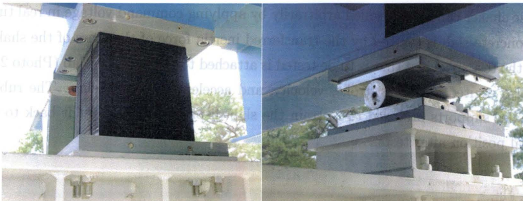
Photo 2.3: Photo of the Rubber and Roller Supports
