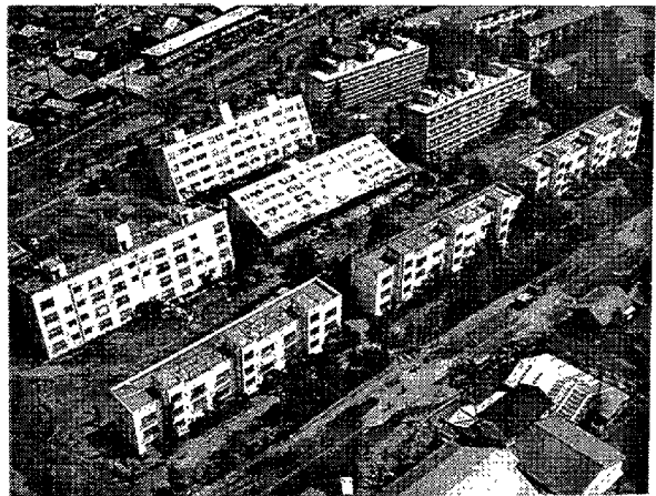
Photo 2 Overturn of Kawagishicho apartment house due to Niigata Earthquake
