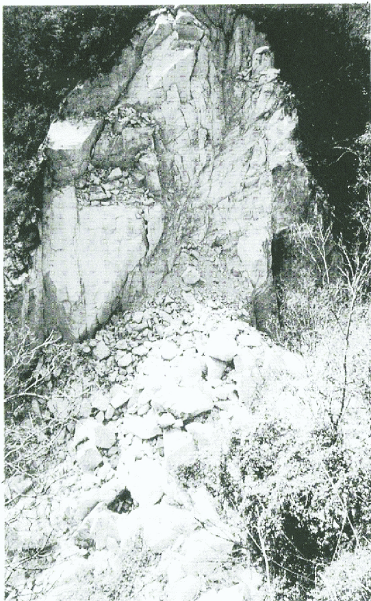
Photo. 1 Failed surface and deposited materials
