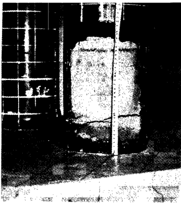
Photo. 3 Failure of filled concrete (1D-pile)
