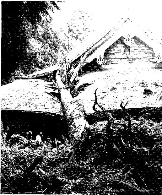
Photo 1 Roof damage by huge tree collapsing from the roof (Syakadou at Heizan Enryakuji-Temple)
