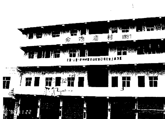
Photo 3 Safety building in the Jingjiang diversion zone (Gongan City)
