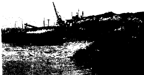
Photo 10 Breach of a dyke at Jiujiang
