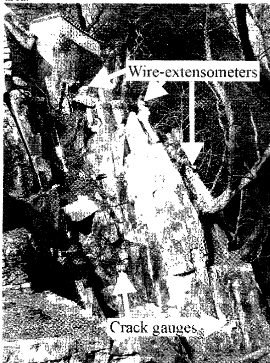
Fig. 6 Photograph of the studied rock slope with installed monitoring devices
