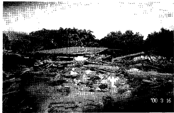
Photo 8 Steel-frame schoolhouses destroyed by flood water accompanied with large amount of driftwood (taken at the place of ④)
