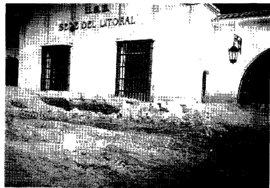
Photo 10 The road facing the entrance gate of the university was deposited about 1 m deep with fine sediments (taken at the place of ⑥)
