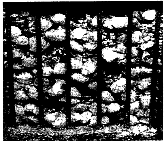
Photo 1 Open spaces blocked by boulders
