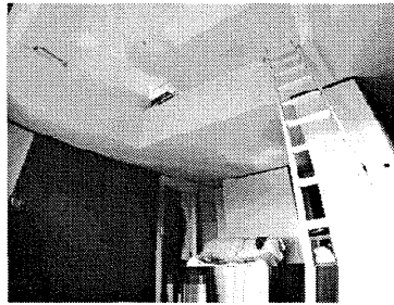
2-501 D2' a (Loft) 電工
