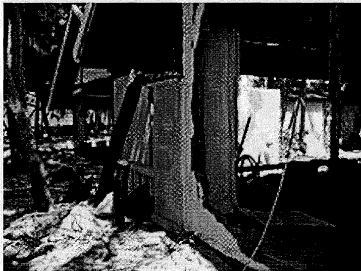
Photo 4.11 The broken wall of a house built of brick in Patong beach
