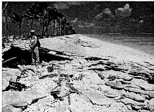
Photo 5.2 Damaged shore protection works
