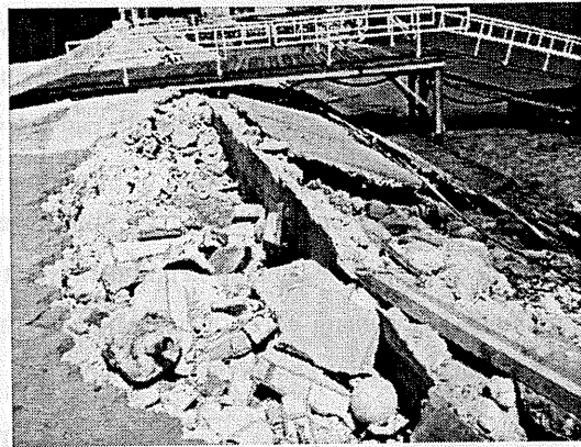
Photo 5.5 Damaged seawall
