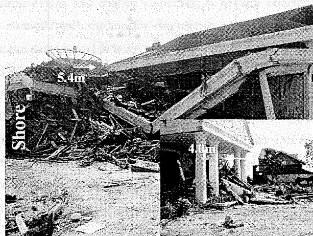
Photo 5 Partially damaged family house located at a distance of about 1.3 km inland from the shoreline in Banda Aceh. Left side is shore and right side inland. Numerals indicate inundation depths.
