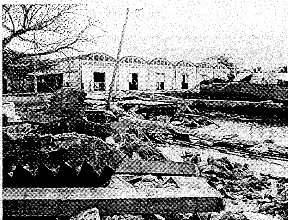
Photo 5 Damage of the quay at the Galle Port
