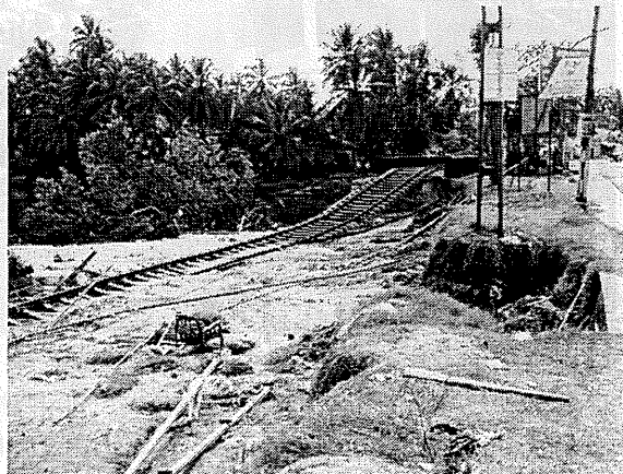
Photo 10 Scouring damage on the foundation of railway at Ambalangoda
