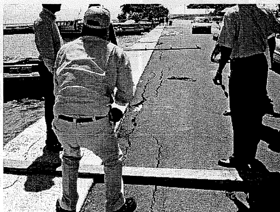
Photo 5.47 Seawall Damage in Fishing Harbour
