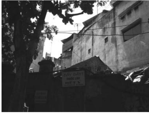
Fig. 6(e) Houses at Point in Fig. 6 (d): A
