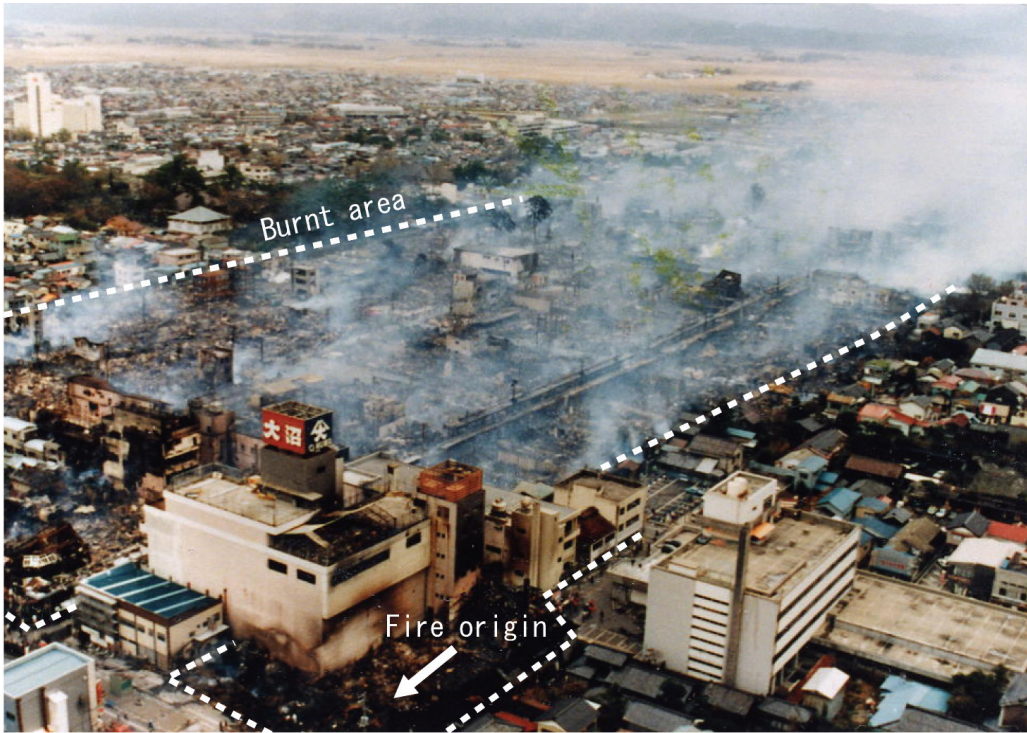
Fig.11. Bird's eye view of the burnt area looking from the west to the east.
