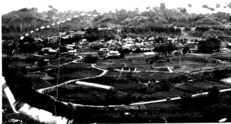
Photo. 3 The view of the Ohkubo landslide taken from the opposite of Chikuma river (on the right side of the river). The enclosed part with the broken line showed the active landslide area.
