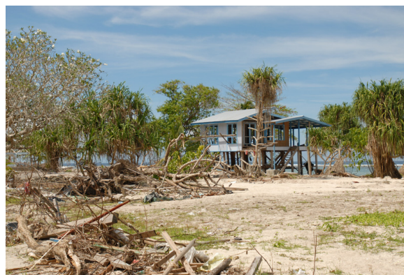
Photo 1 Damage at Titiana Village (May 27, 2007)
