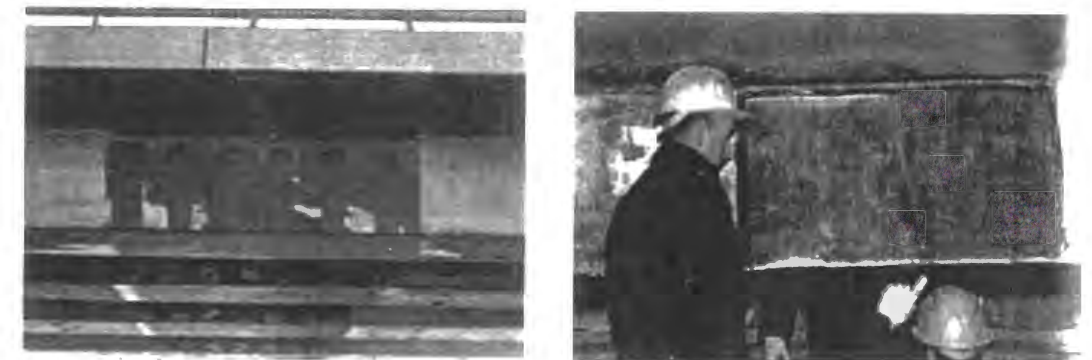
Figure 2.6 FRP retrofitting for shear
