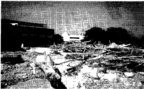
Photo 7 Sediment and driftwood deposited at the school building. The reinforced concrete building was buried one floor deep with sediment (taken at the place of ③)
