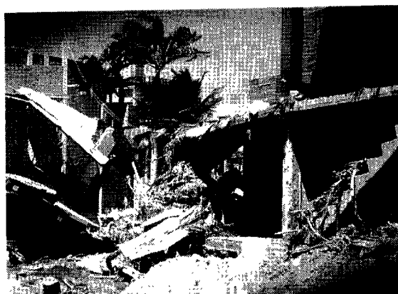
Photo 4 Damaged slum quarters
