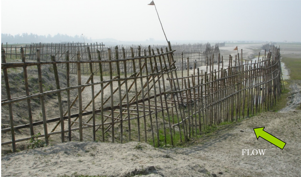
Photo 4.1 Bandal-like structures for river channel stabilization at Jamuna river – Bangladesh (January, 2010) – upstream side view
