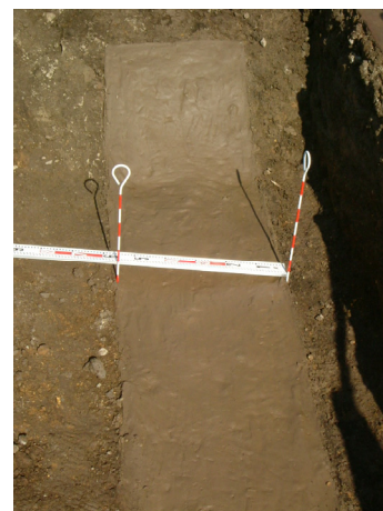
Photo 1.2 Appearance of SBM cutoff wall after construction.
