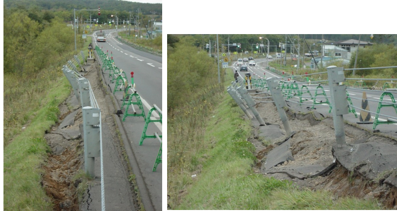
Figure 5.2 Shallow sliding failure in a road embankment in Chokubetsu, Onbetsu-cho during the 2003 Tokachi-oki Earthquake, Hokkaido, Japan (Yoshimine, 2003)
