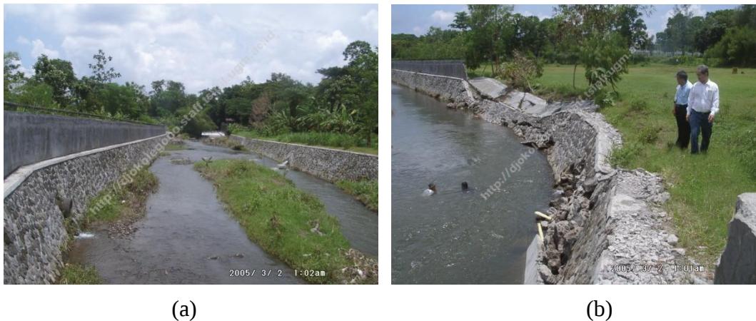
Photo 1.1 Failed structure at outer bank. (Photo courtesy: Djoko Legono)
