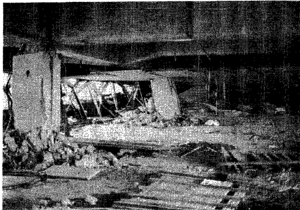
Photo. 2 Mutsu City Office Building
