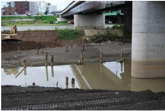
Photo 4 Former wood pile foundations near Kida Bridge
