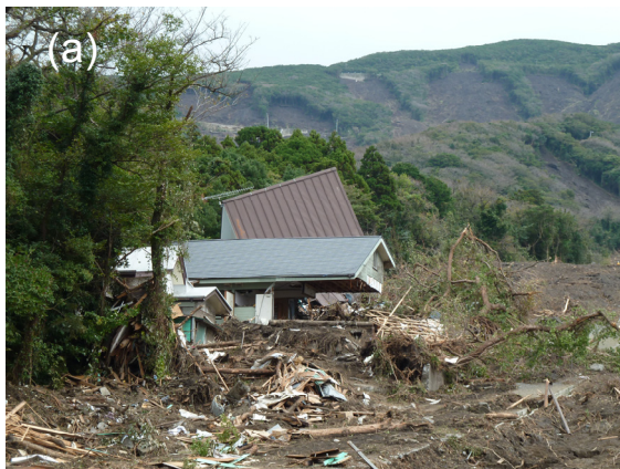
Photo 1 Residential and physical damages by sandy-muddy debris flows subsequent to the shallow landslides
