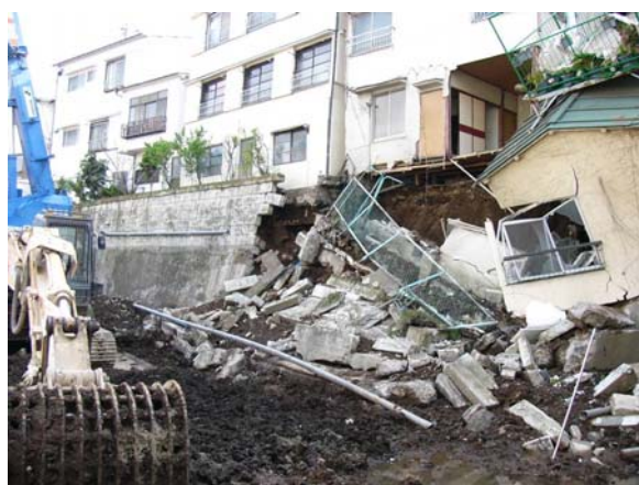
Photo 3 Collapse of small residential fill in Tokyo, 2004
