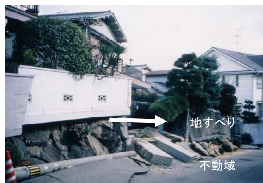
Photo 2 Landslide in residential valley fill in Nishinomiya City, caused by the 1995 earthquake
