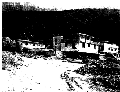
Photo 6 Damaged houses in Uria
