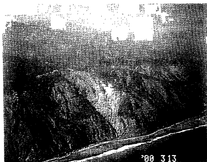
Photo 1 Densely distributed landslides on the hill slopes near coastal line
