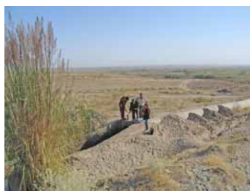
Fig. 2.6 Head-water intake infrastructure passing into earth Muminov' channel
