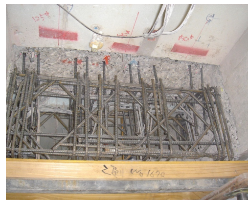
Photo 7 A strengthening work for a building intentionally false designed by Aneha
