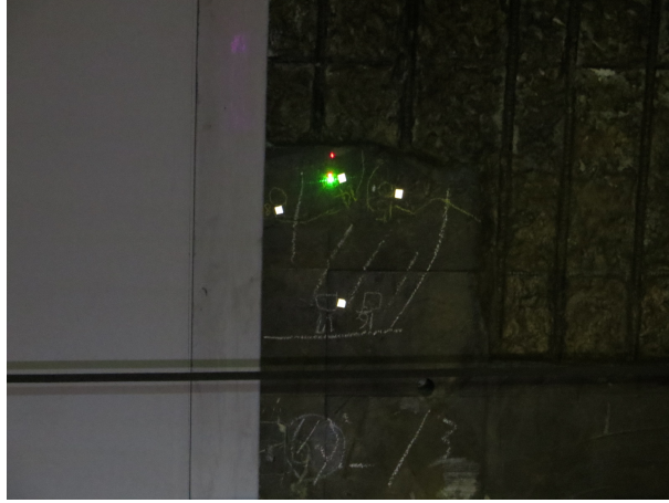
Figure 20: Tunnel lining around experiment location 3.
