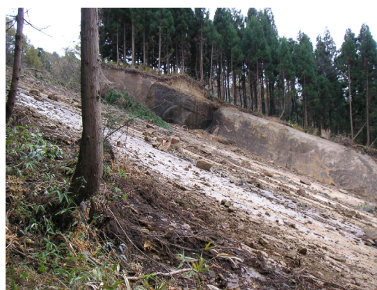
Photo 2 Slope collapses at Yokowatari area. (enlarged photo)
