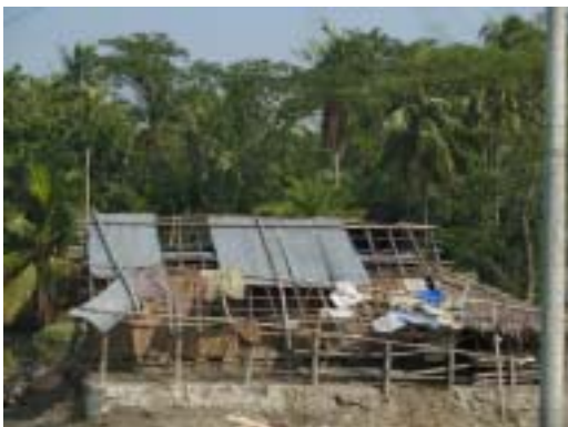
Fig.3 Damaged house in Sharankhola
