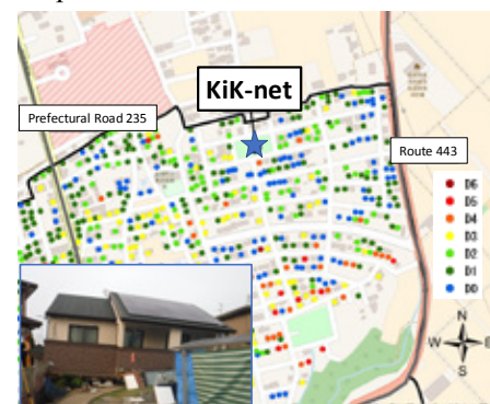
Figure 3. Collapsed building near the KiK-net station.
