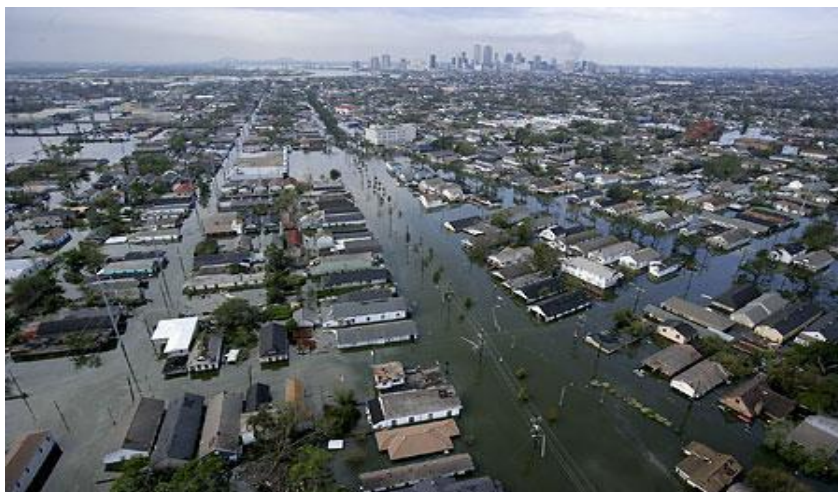
Figure 1.12 Inundation disaster of downtown at New Orleans, United States (Photo Courtesy: MLIT, Japan)
