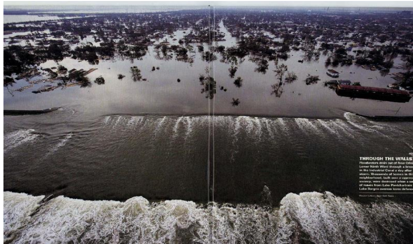
Figure 1.13 Inundation disaster by dyke failure at New Orleans, United States (Photo Courtesy: MLIT, Japan)
