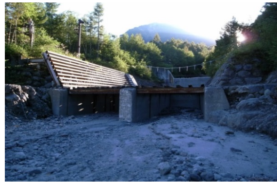
(b) Debris-flow breaker in Japan
