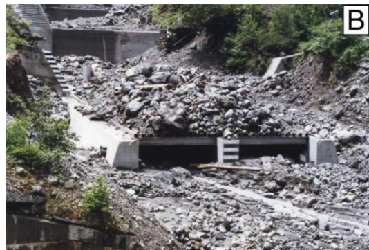
(b) Boulder deposits of the July 21, 1985 debris flow trapped on the breaker (Photo taken July 22, 1985)
