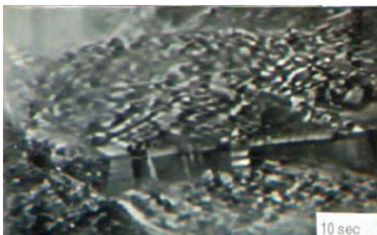
Photo 2.2 Debris-flow breaker stopping the front portion of a debris flow
