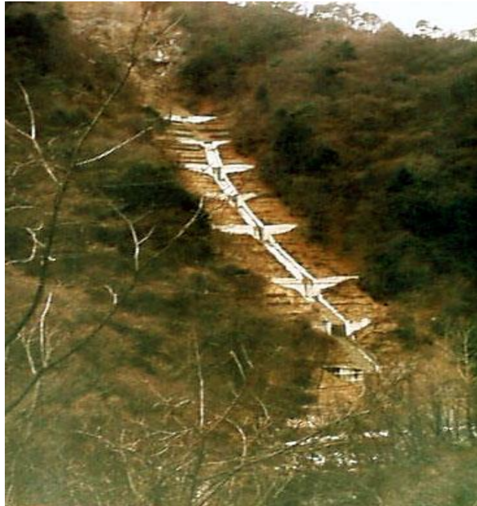
(a) A series of Sabo dams in Nagano Prefecture
