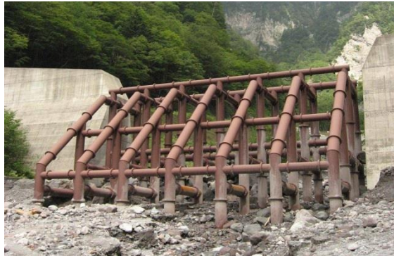
(a) Grid Sabo dam in Gifu Prefecture, Japan (Data source : Shresta et al., 2008)
