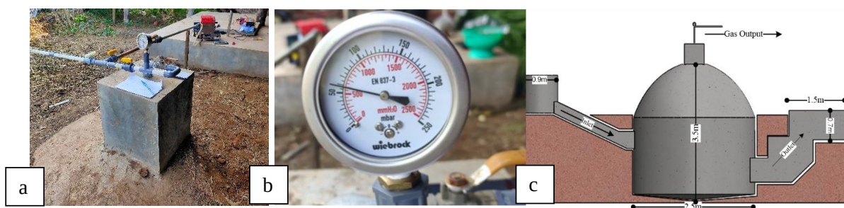
Figure 5.7 (a) Unit digester, (b) gas pressure, and (c) sketch of unit
